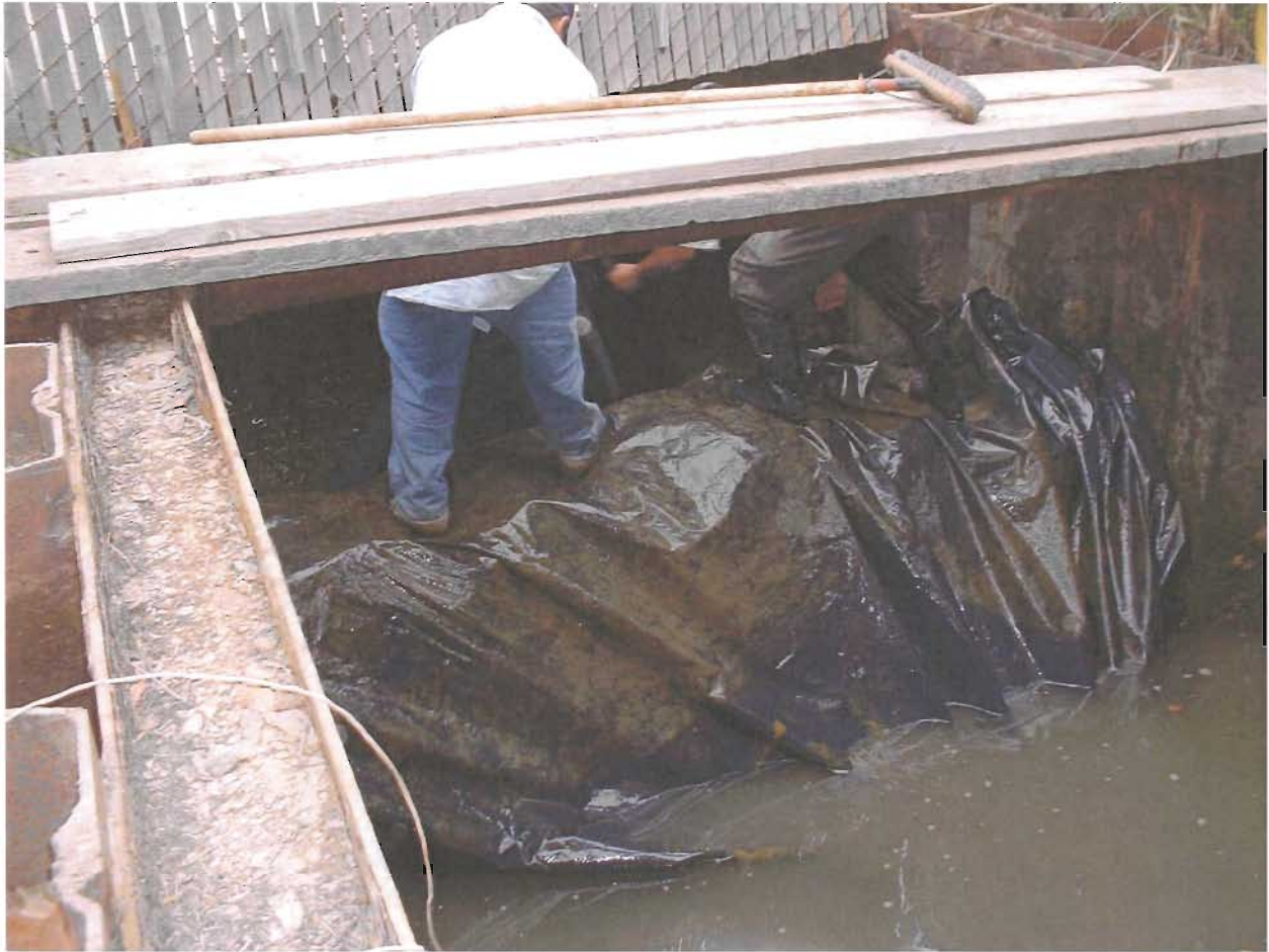
Figure 2 - Temporary tide barrier installation before the infiltration test.
