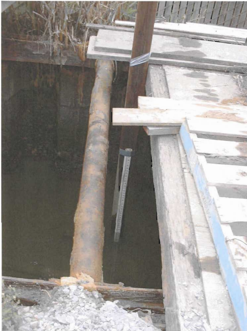
Figure 3 - Measurement of change in water level upstream of the temporary tide barrier.
